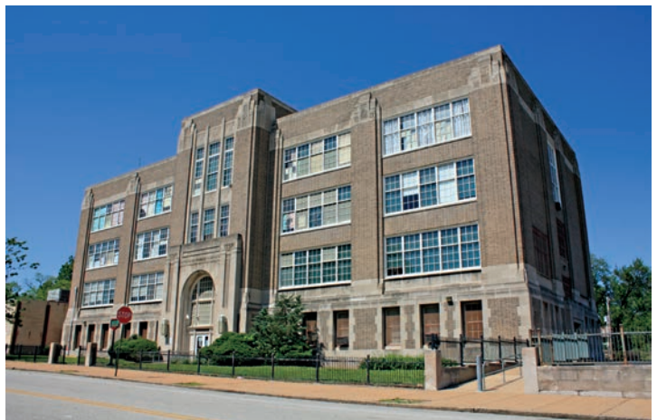
Cole Elementary School, 3935 Enright Ave Photo by Chris Naffziger, 2016
