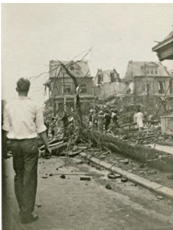
Tornado Damage to 4201 Westminster, by unknown, 1927. Courtesy Missouri Historical Society, P0981-0000.
