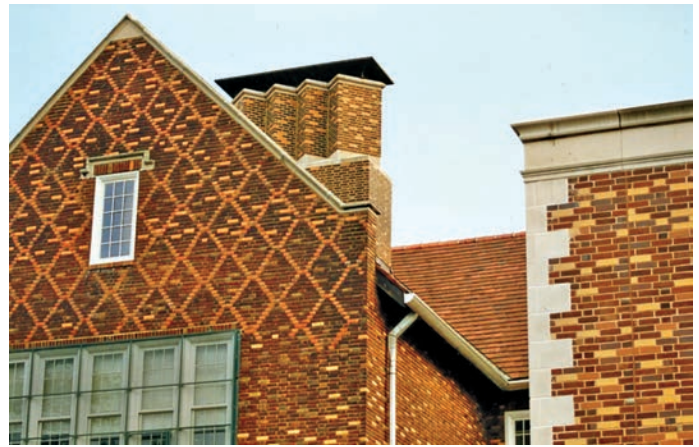
The use of cull bricks adds visual interest.
