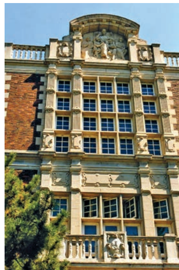
The grand entry façade of Soldan High School
