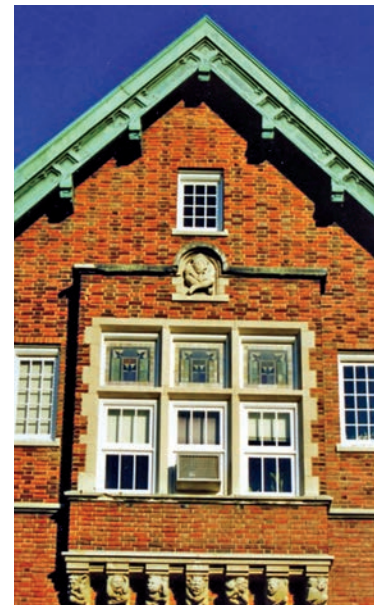
Shepard school. Note the detailed stone window surrounds, the brick patterns and the carved stone figures.
