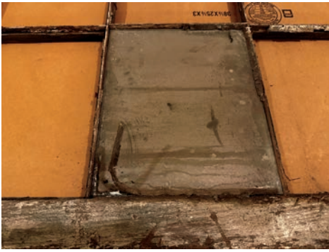
The original glass pane in the window frame before being cleaned
